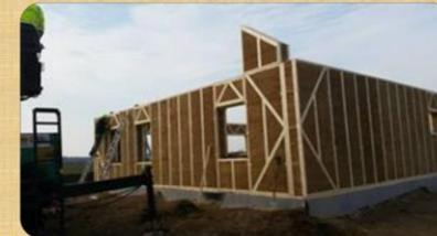
Fig.1 Frame system with straw panels
